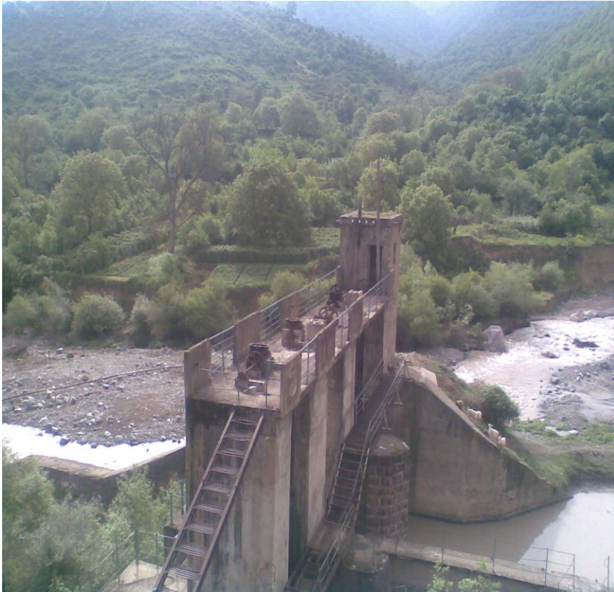
Water intake facility of Zurnabad HPP Gancachay river
